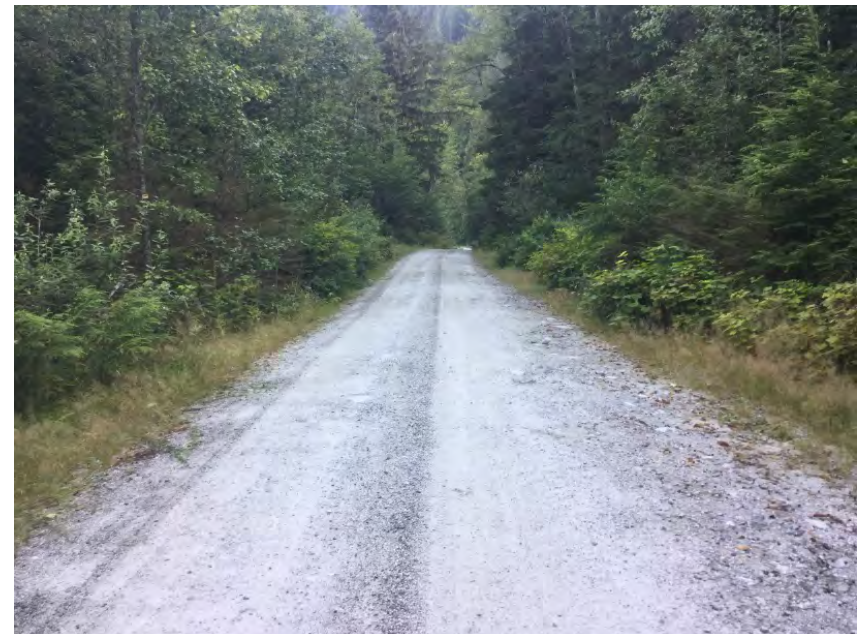
Right Approach Facing Away From Culvert
