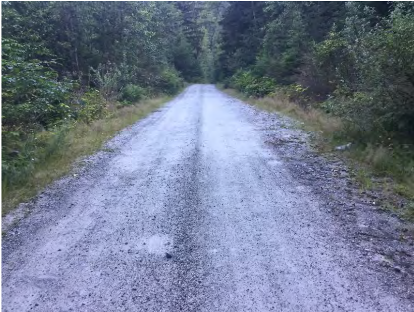
Left Approach Facing Culvert
