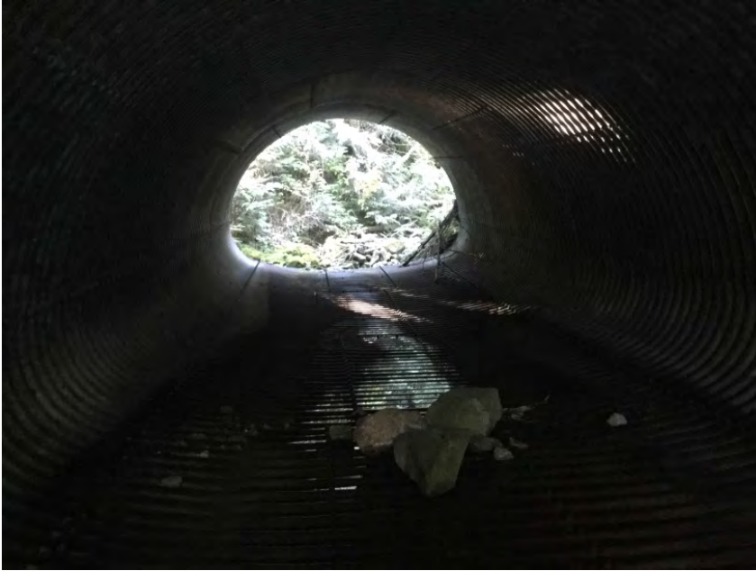
Barrel of Culvert 1
