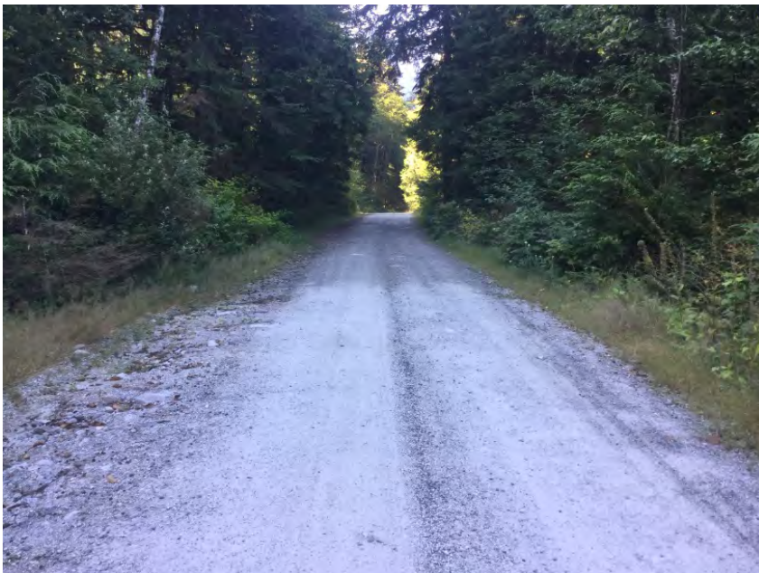
Left Approach Facing Away From Culvert
