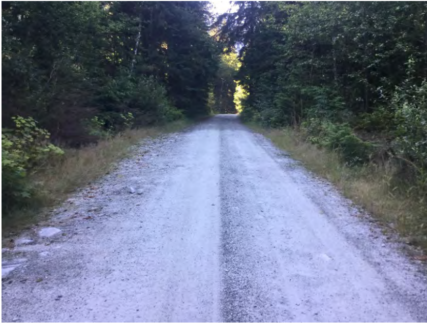
Right Approach Facing Culvert
