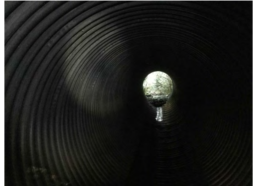
Barrel of Culvert 2
