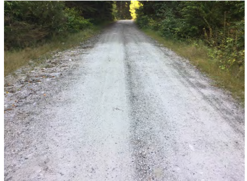
Roadway Over Culvert
